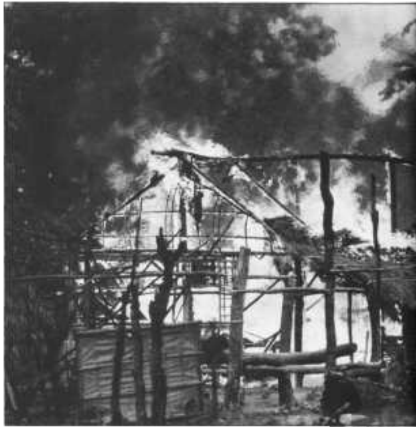
Scorched earth: Destruction caused during a Khmer Rouge retreat
