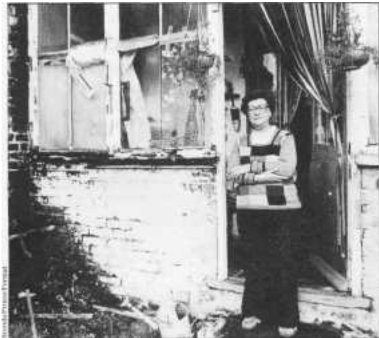
Rising damp and falling expectations
