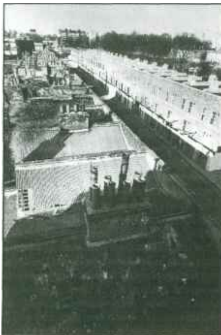
Council refurbishment, London
