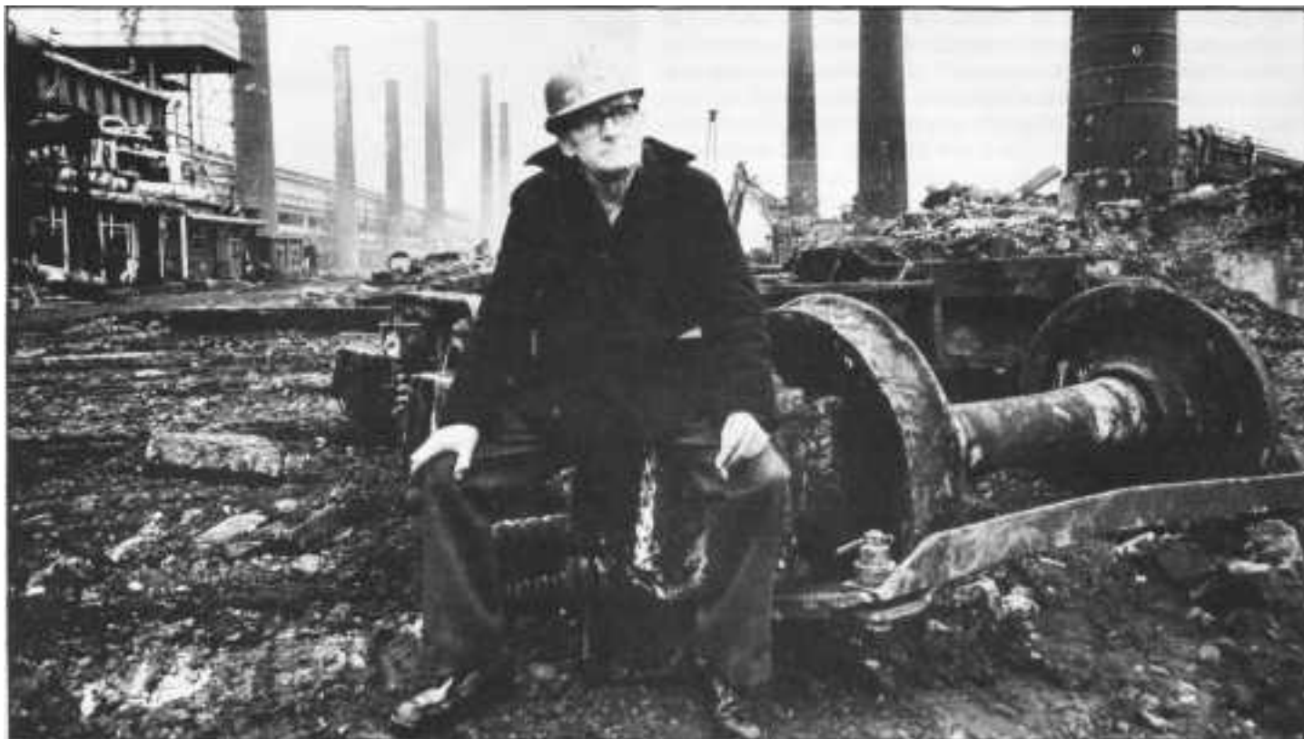
A man who has spent all his working life at East Moors steelworks in Cardiff is now employed to help demolish it
