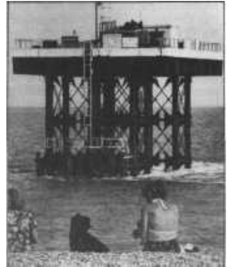
Offshore water outlet at Sizewell
