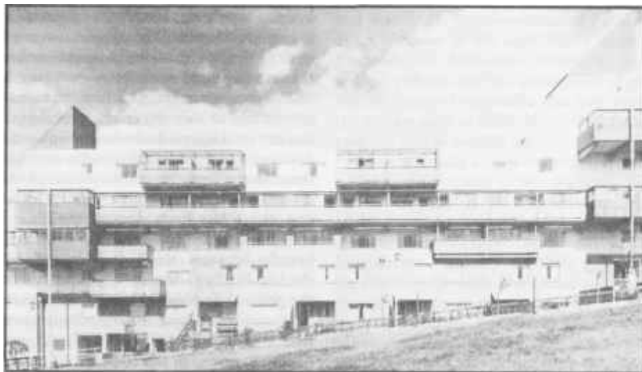
New housing at Byker, Newcastle. One of the last of the big redevelopment schemes and one of the best.
